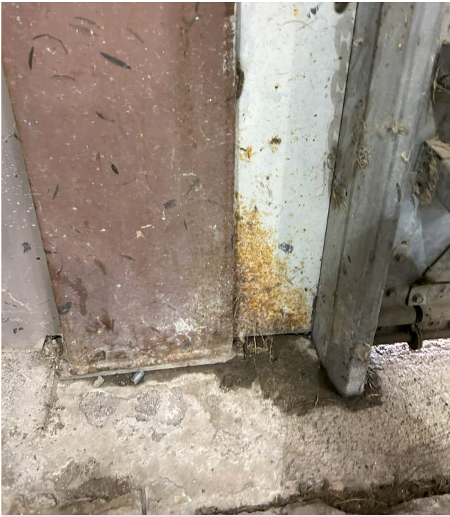
MOISTURE INTRUSION AT BASE OF WALL
