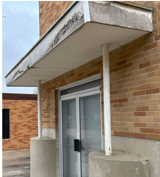
FAILING ENTRY CANOPY
