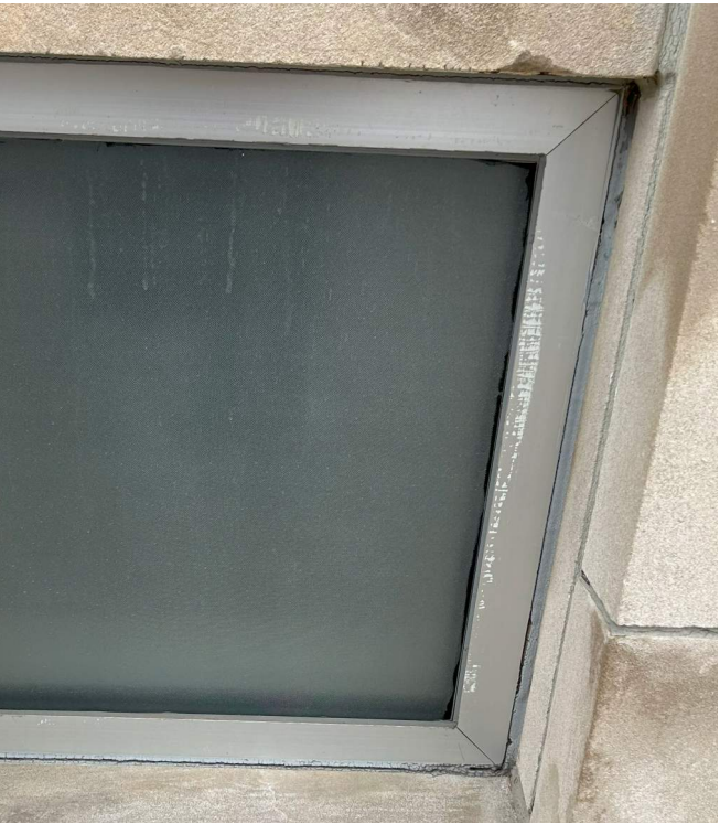
NON THERMALLY BROKEN FRAMES AND SINGLE PANE GLAZING
