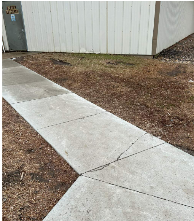
SIDE WALK CRACKING
