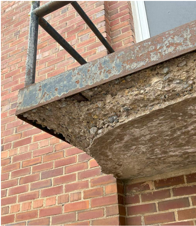
FAILING LANDING AT EGRESS STAIR
