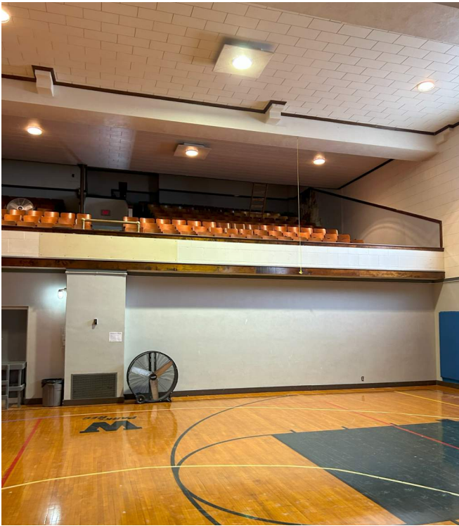
ACOUSTIC CEILING PADS - TYPICALLY ASBESTOS CONTAINING MATERIAL
