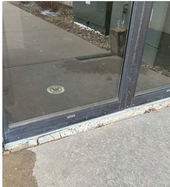
NO STOOP AT EXTERIOR/ALUMINUM FRAME
