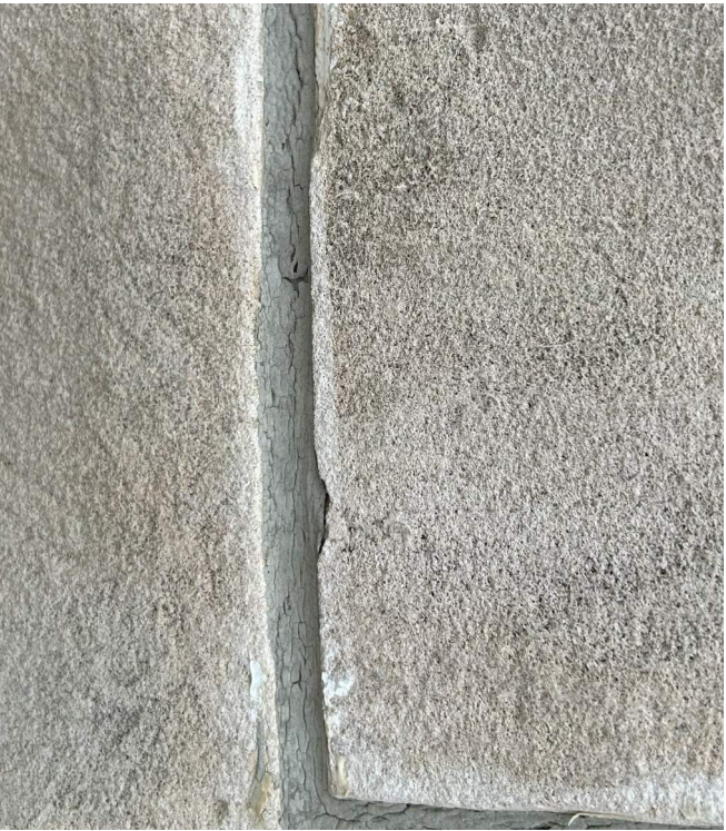
DRY ROT/FAILED SOFT JOINTS AT LIMESTONE
