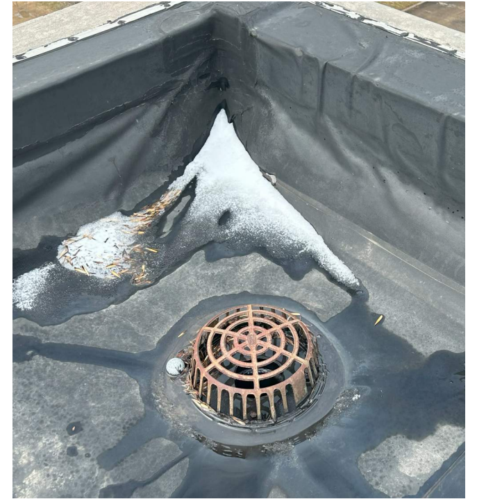
MEMBRANE DELAMINATION AT PARAPETS
