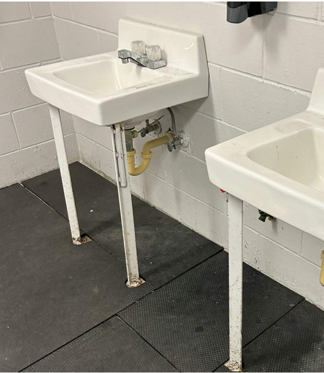
NON-ADA COMPLIANT FIXTURES
