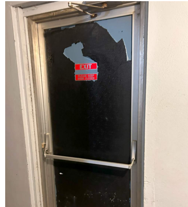
1980s ALUMINUM FRAMES AND FAILED PANEL
