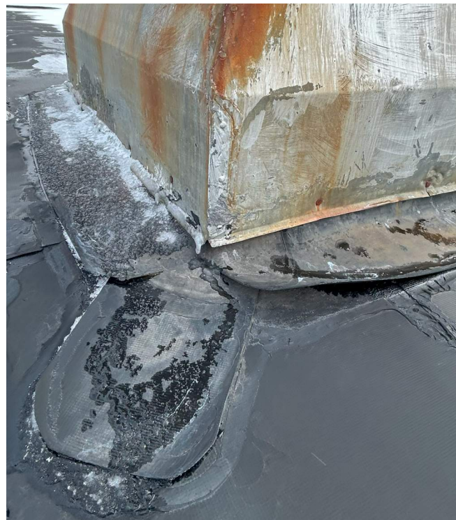
SEAM DELAMINATION AT ROOF PENETRATIONS
