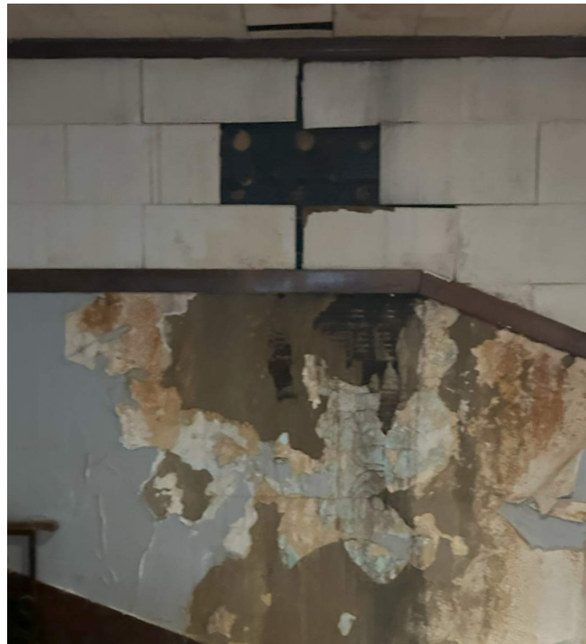
MOISTURE INTRUSION AT ROOF LEAKING
