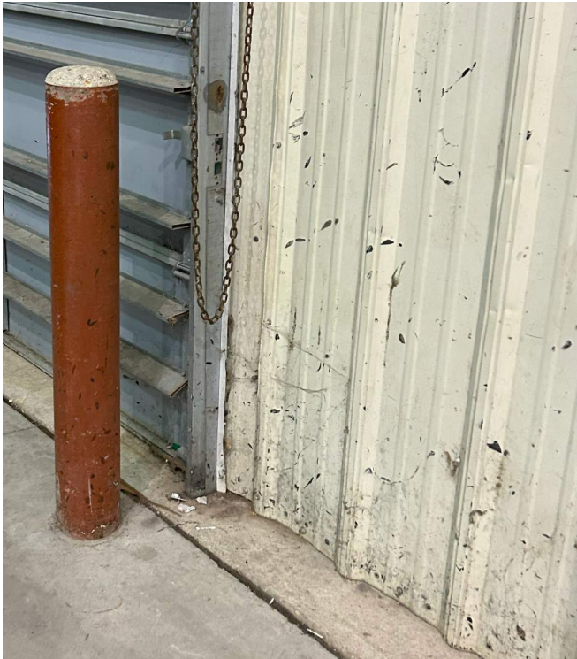
PUCK DAMAGED INTERIOR LINER PANEL
