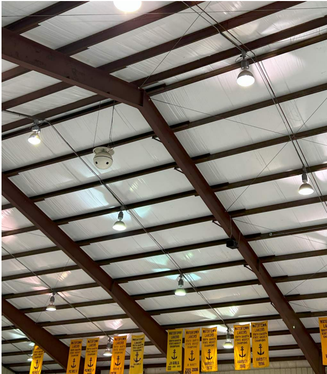
METAL BUILDING ROOF INSULATION
