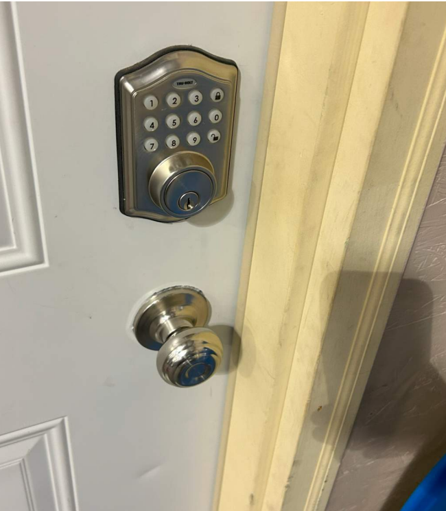
NON ADA COMPLIANT DOOR HARDWARE
