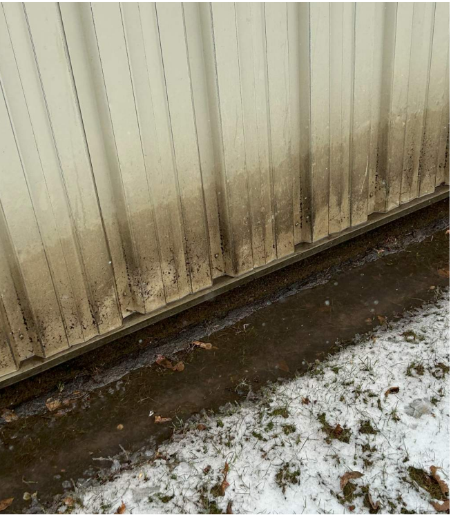
BASE OF WALL WATER DAMAGE
