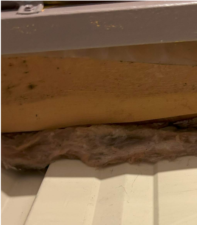
INSULATION DAMAGE AT LEAN-TO TIE IN
