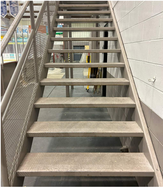
OPEN RISERS, NO HANDRAILS
