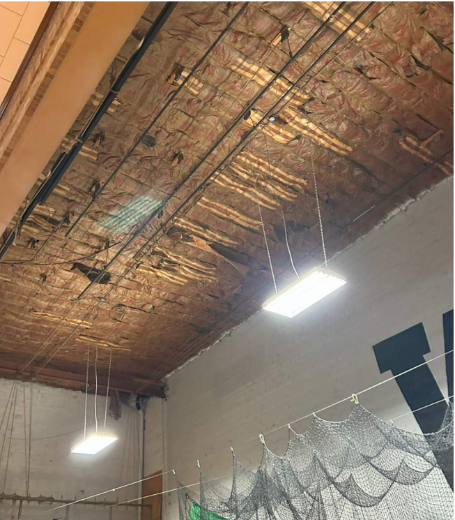
WAX COATED, KRAFT-FACED BATTING
