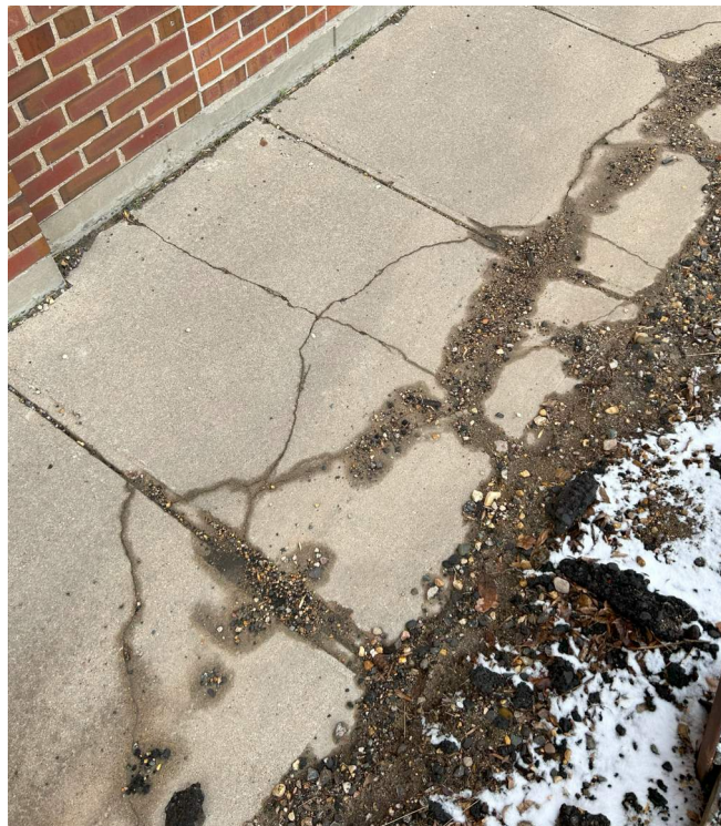
CRACKED WALKWAYS AT NORTH PARKING
