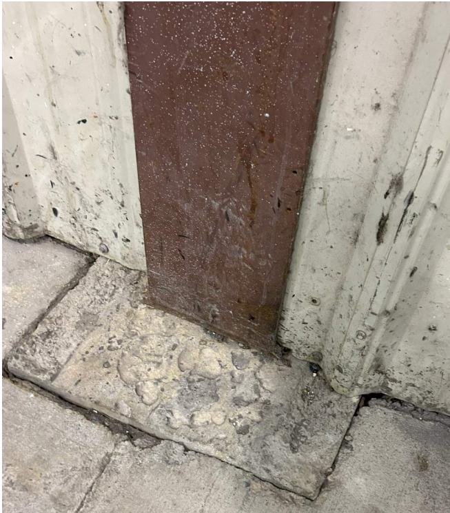
PEMB COLUMN BASE - TYPICAL
