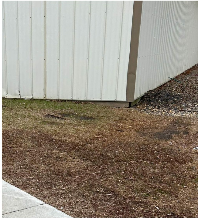
LEAN-TO BUILT ON WOOD SKID
