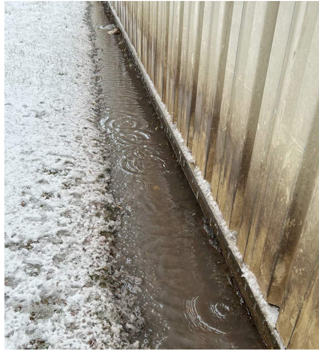
NO WATER CONTROL AT BUILDING PERIMETER
