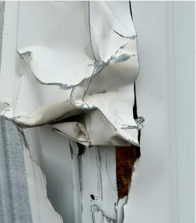
DAMAGE AT EXTERIOR METAL WALL PANEL
