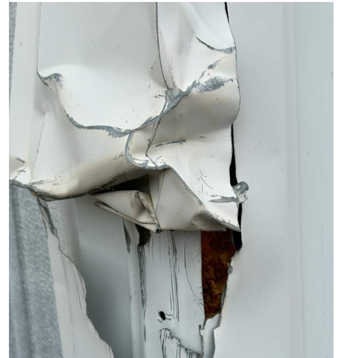
DAMAGE AT EXTERIOR METAL WALL PANEL
