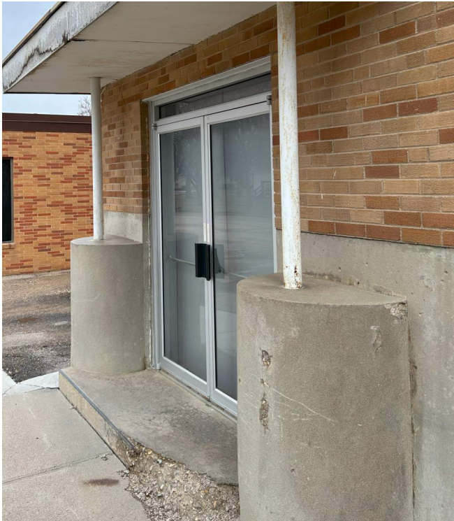
INACCESSIBLE ENTRANCES/SPALLING STOOP
