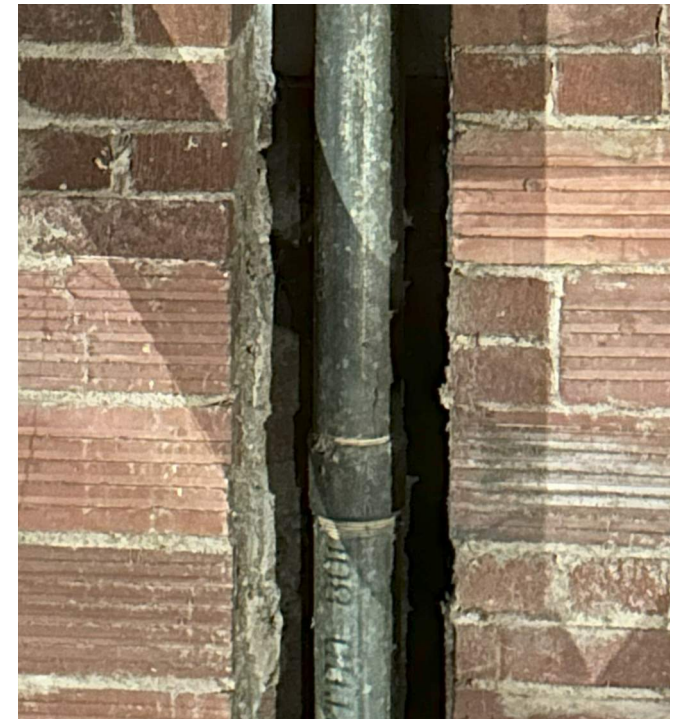
COMPROMISED STRUCTURE AT BATHROOM VENT
