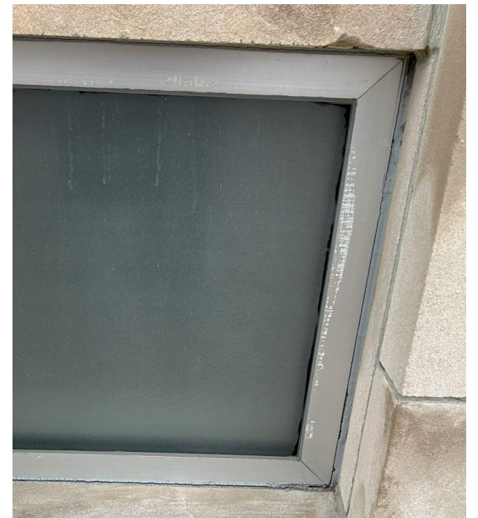
NON THERMALLY BROKEN FRAMES AND SINGLE PANE GLAZING
