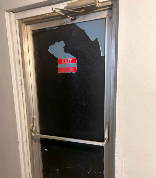
1980s ALUMINUM FRAMES AND FAILED PANEL
