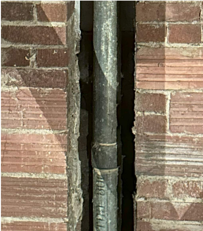
COMPROMISED STRUCTURE AT BATHROOM VENT
