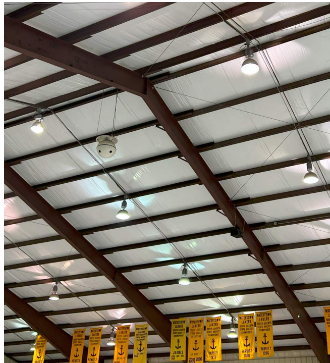
METAL BUILDING ROOF INSULATION
