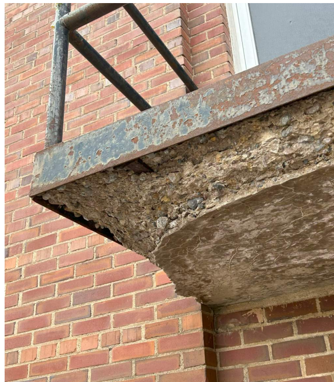
FAILING LANDING AT EGRESS STAIR
