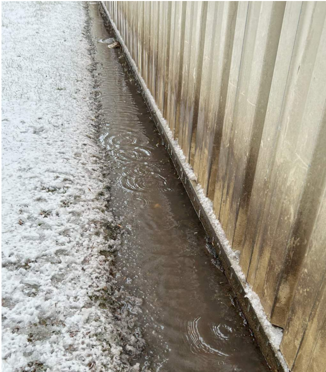
NO WATER CONTROL AT BUILDING PERIMETER
