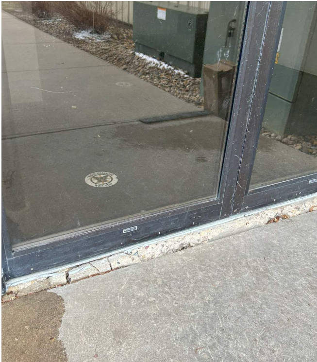
NO STOOP AT EXTERIOR/ALUMINUM FRAME
