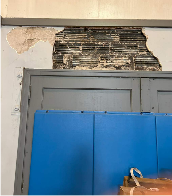
DAMAGE AT GLASS BLOCK LEAK
