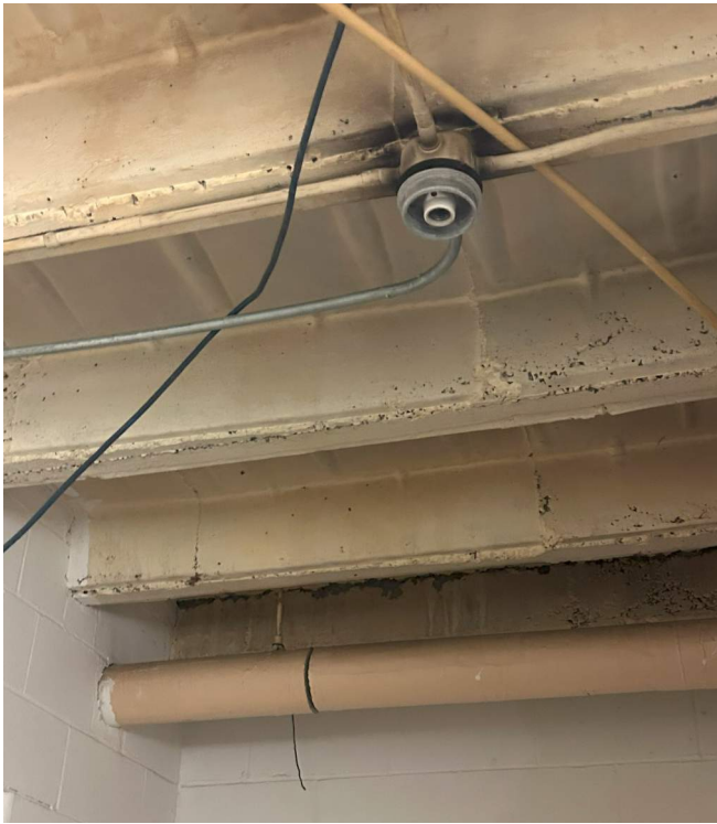
CONCRETE PAN FLOOR - GOOD CONDITION
