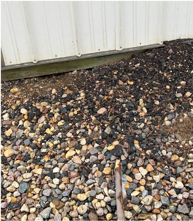
GRADING OVER FIRST FLOOR LEVEL
