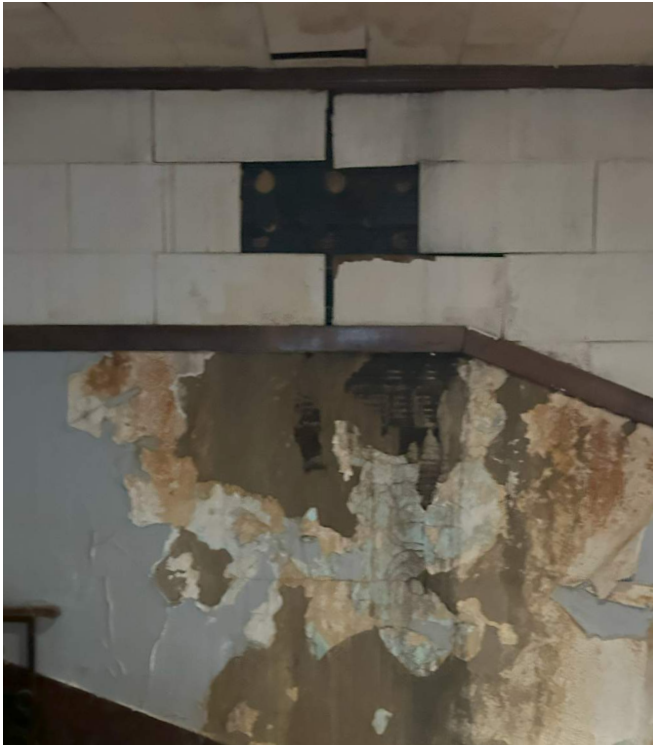
MOISTURE INTRUSION AT ROOF LEAKING
