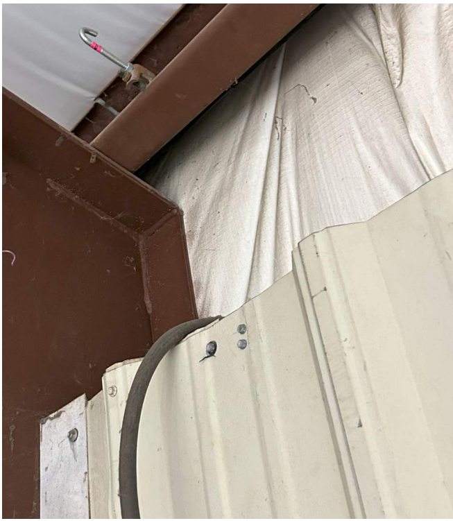
SIMPLE SAVER WALL INSULATION - GOOD CONDITION
