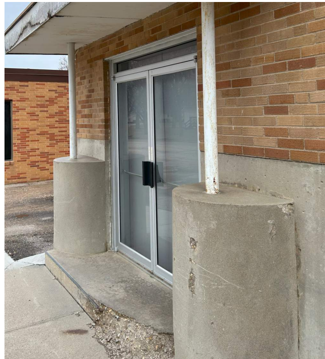
INACCESSIBLE ENTRANCES/SPALLING STOOP
