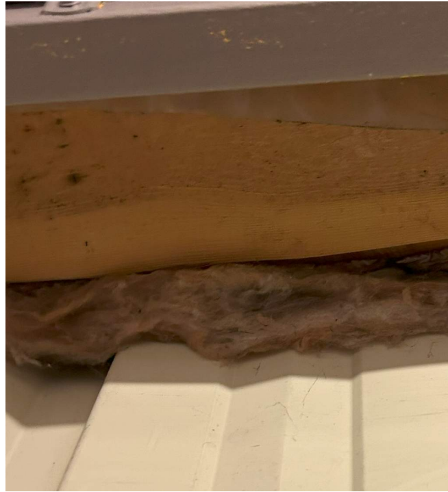
INSULATION DAMAGE AT LEAN-TO TIE IN
