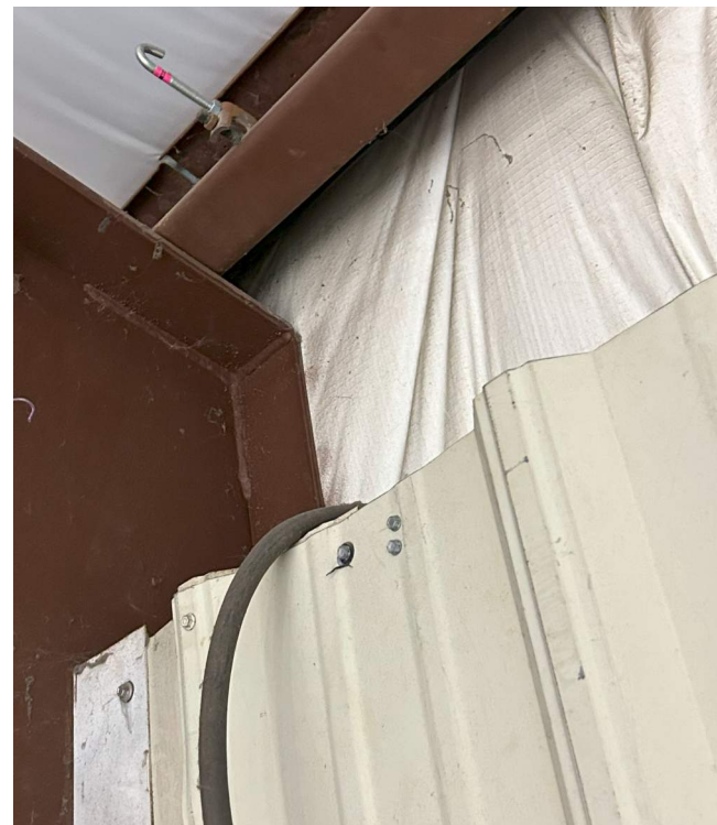
SIMPLE SAVER WALL INSULATION - GOOD CONDITION
