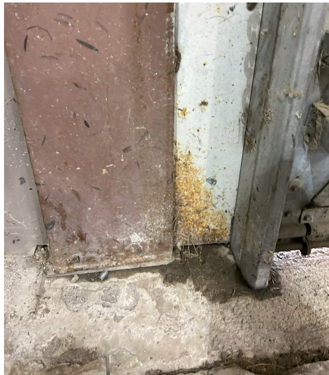
MOISTURE INTRUSION AT BASE OF WALL
