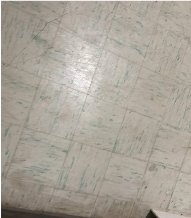
9"X9" RESILIENT TILE - TYPICALLY ASBESTOS CONTAINING MATERIAL
