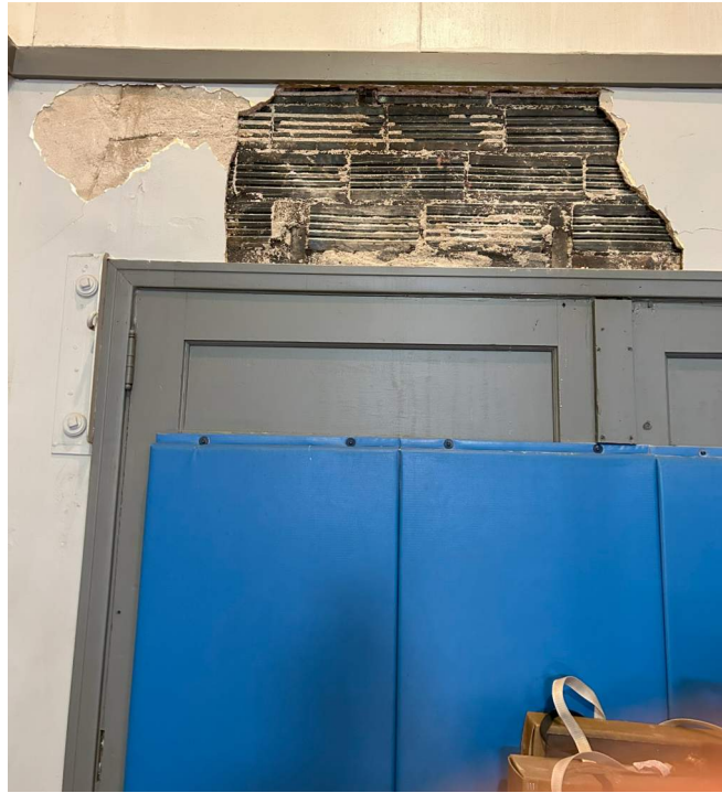
DAMAGE AT GLASS BLOCK LEAK
