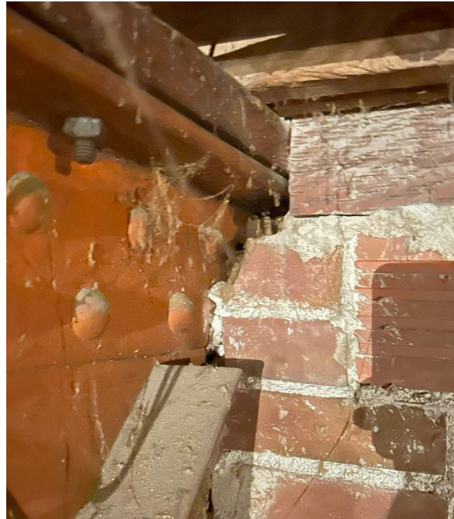
TRUSS CONNECTION AT EXTERIOR WALL
