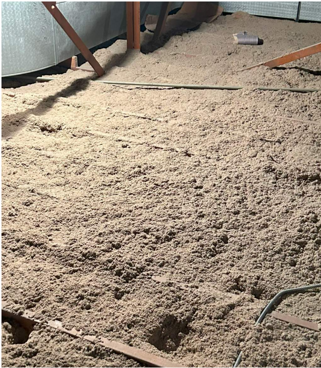
BLOWN CELLULOSE INSULATION AT ATTIC
