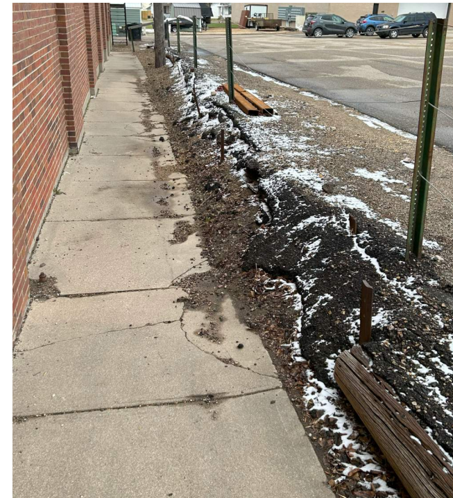
POOR DRAINAGE/BAD FENCE AT PARKING LOT
