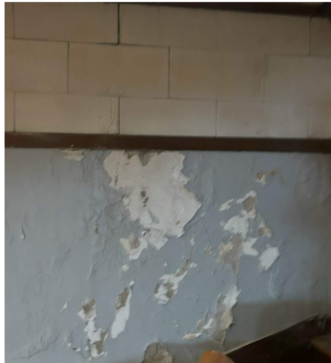
MOISTURE INTRUSION AT ROOF LEAKING
