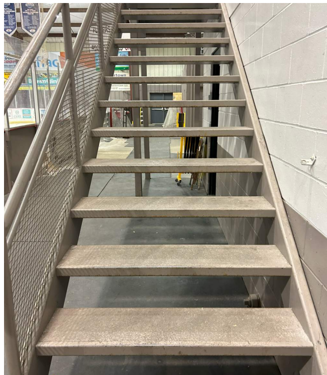
OPEN RISERS, NO HANDRAILS
