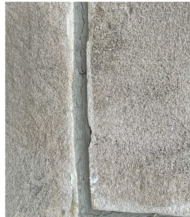
DRY ROT/FAILED SOFT JOINTS AT LIMESTONE
