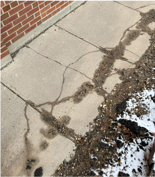
CRACKED WALKWAYS AT NORTH PARKING
