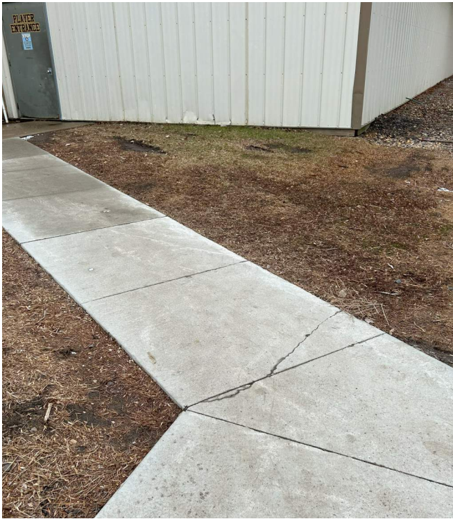
SIDE WALK CRACKING
