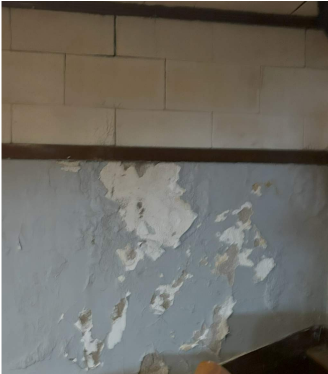
MOISTURE INTRUSION AT ROOF LEAKING
