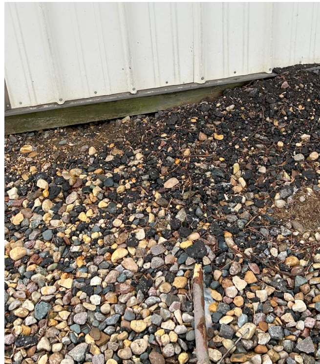
GRADING OVER FIRST FLOOR LEVEL
