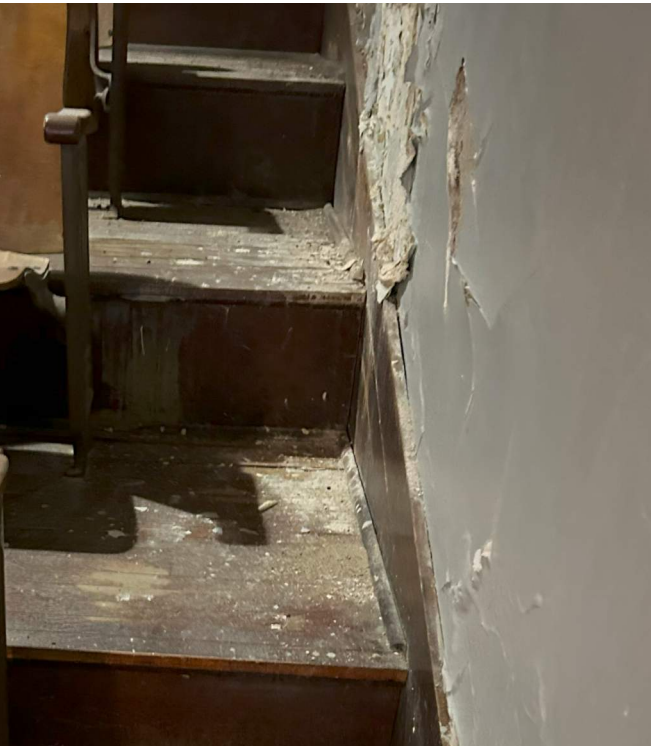
DAMAGED RISER FLOORING AT ROOF LEAK
