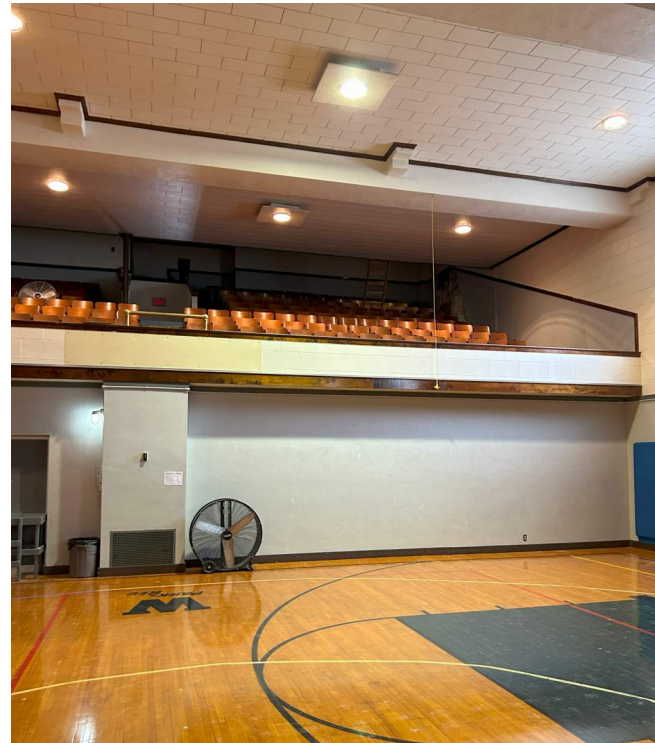
ACOUSTIC CEILING PADS - TYPICALLY ASBESTOS CONTAINING MATERIAL
