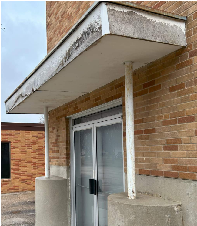
FAILING ENTRY CANOPY
