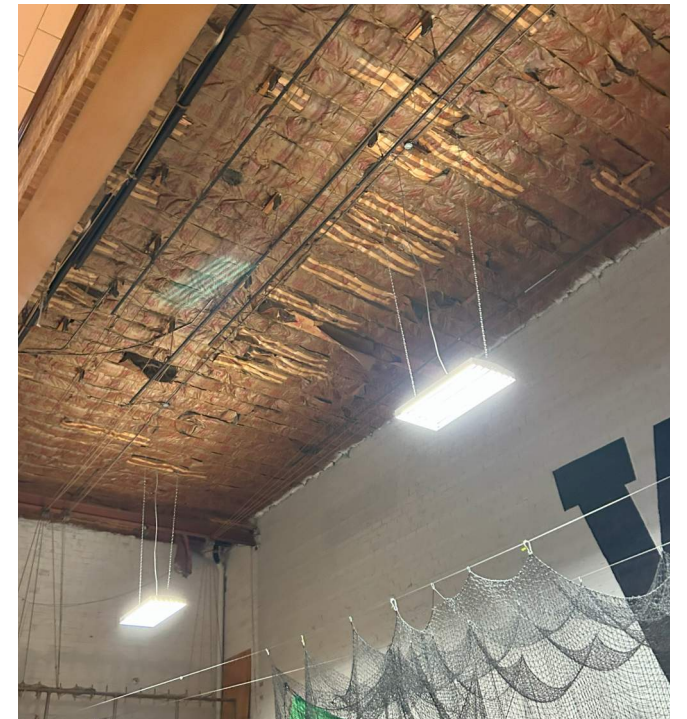
WAX COATED, KRAFT-FACED BATTING
