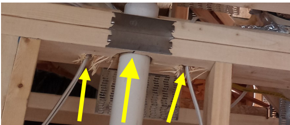
Examples of Fire Blocking needing to be added between the wall and ceiling.
