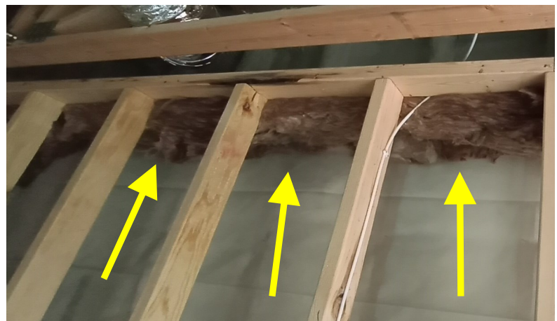
Example of Fire Blocking of furred out wall and ceiling using batts of insulation.
