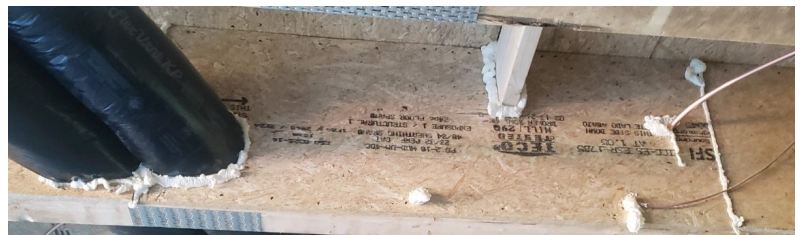
Example of Draft Stopping of a floor truss.
